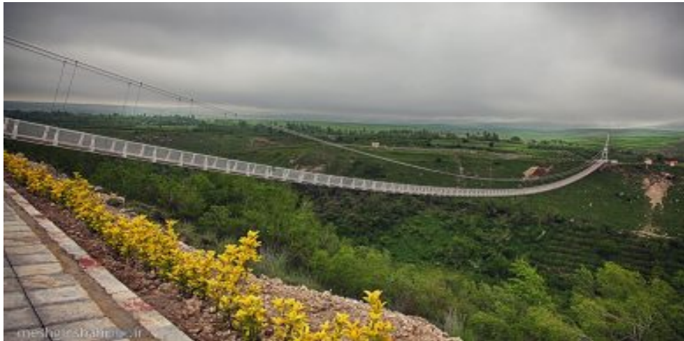
Figure 1. Suspension Bridge in Meshginshahr, Ardabil.
